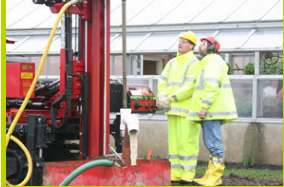
Gateway President Bryan Albrecht and instructor Tom Niesen begin to drill the first hole on the Kenosha Campus to demonstrate the college's new geothermal program. For more information, call Tom Niesen at (262) 564-2610
