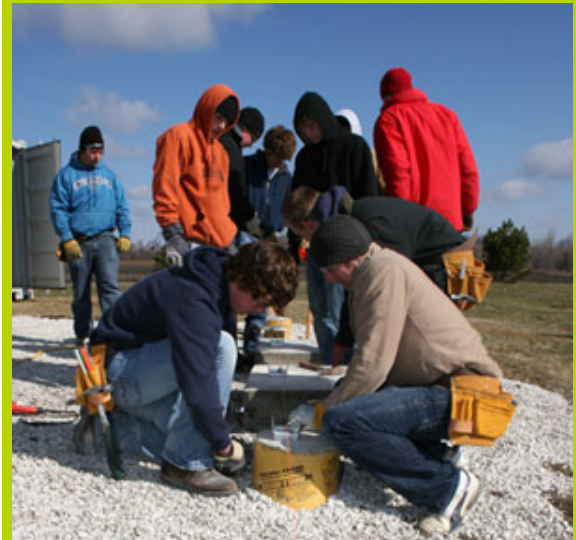
Students and community partners help work on a roof vent prop training deck.
