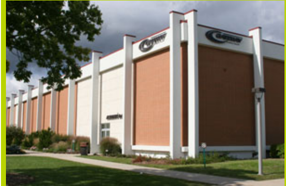
Gateway is in the process of installing new building-mounted, backlit signage to enhance students' and visitors' Gateway experience.
